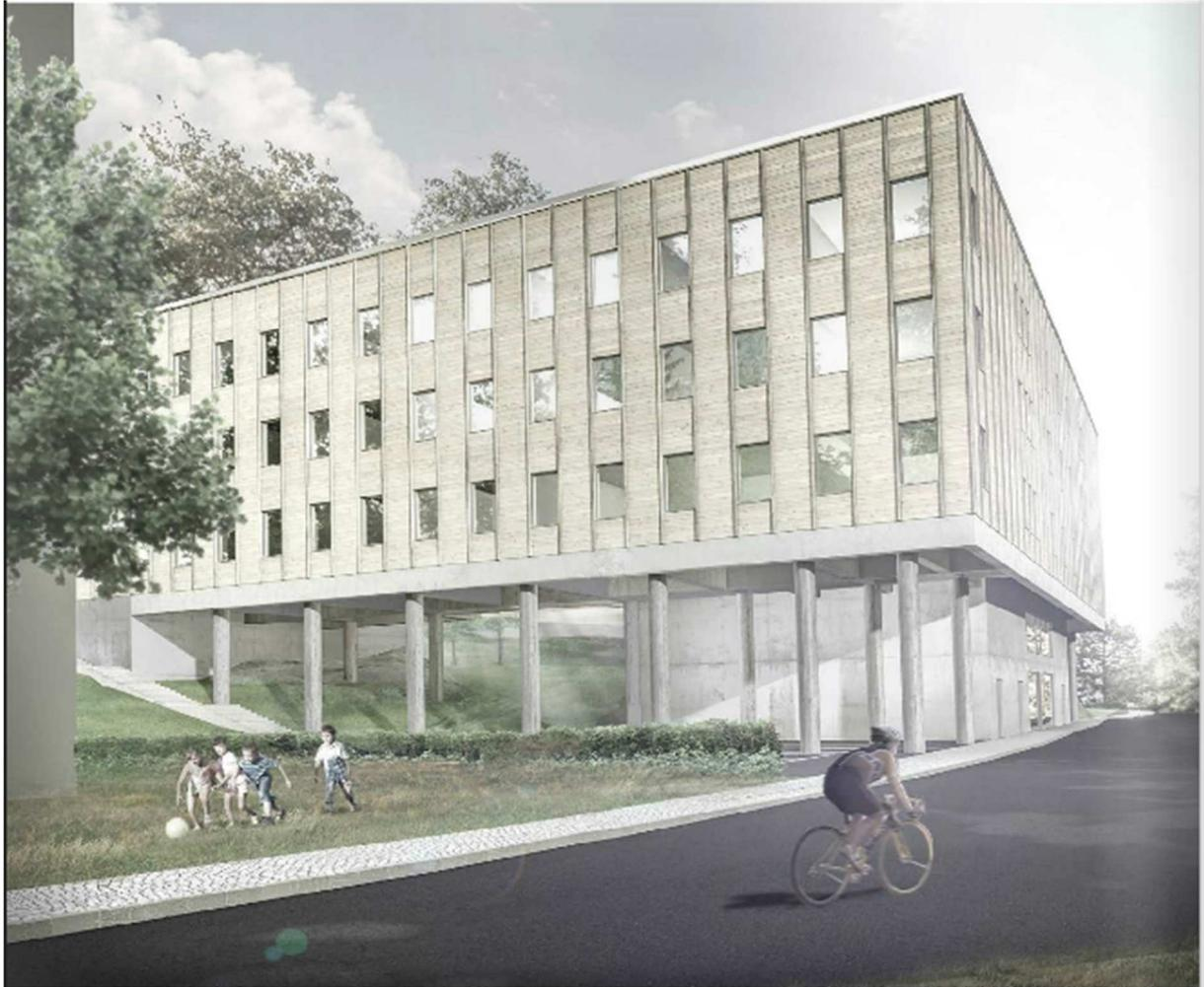
*The U-shaped house's first two floors have a prefab frame in concrete and also include an entrance, RTU and library. The upper floor of the nursing home consists of wooden modules with apartments, a kitchenette and a bathroom. illustration; SR-K (Scott Rasmusson-Källander)*
