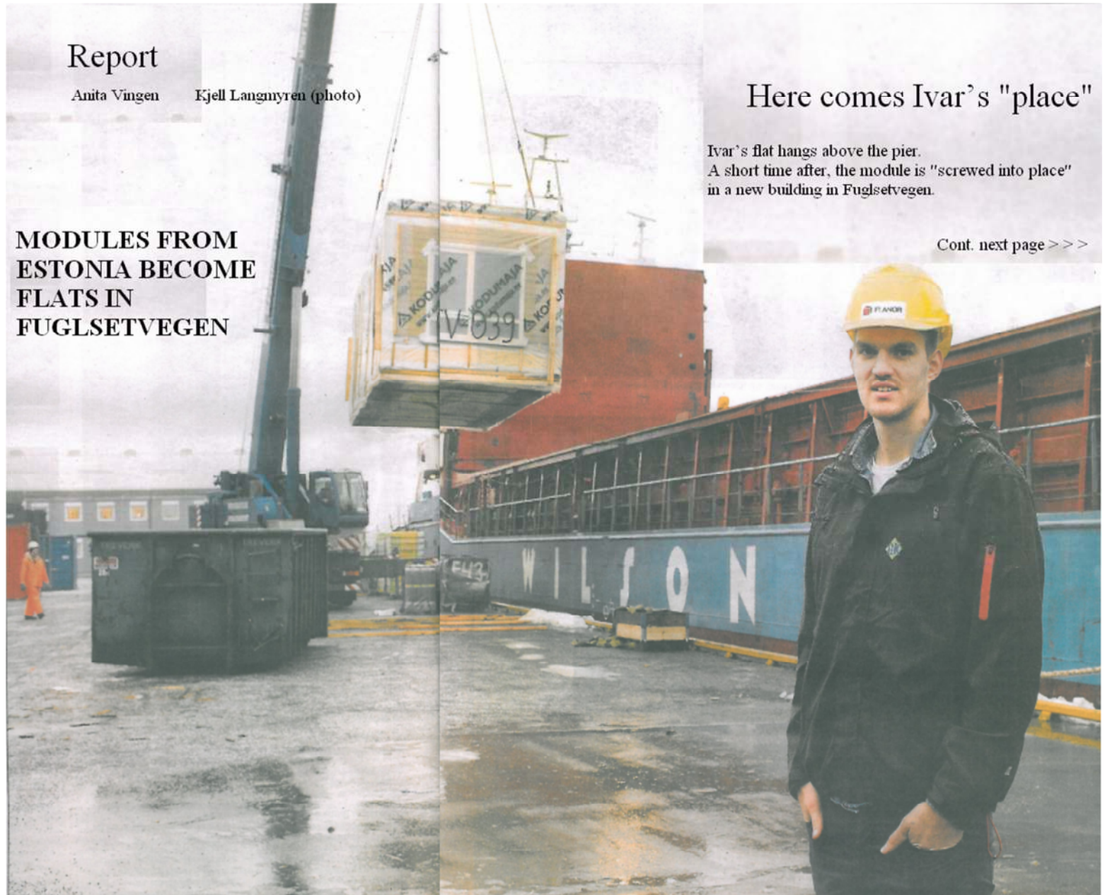
Logistics: After five days of transport from Tallinn to Molde, a whole block of flats is being unloaded. Module after module is lifted from the ship's hold – here is No. 039, which will be half of Ivar Brovold's flat.
